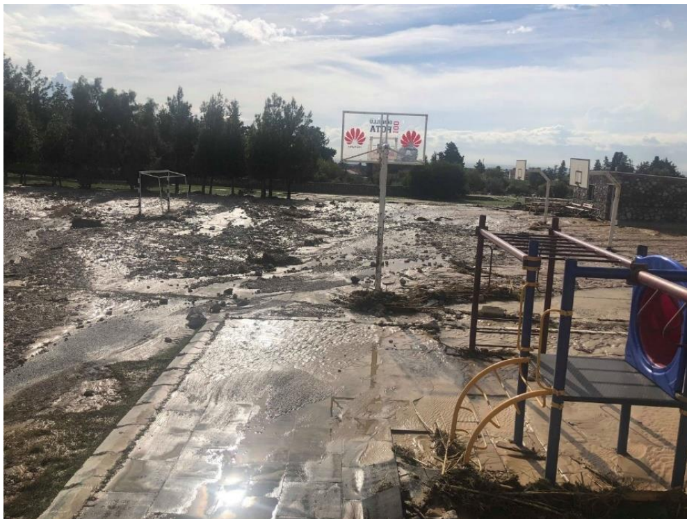
Figure 1.7 Dikmen Primary School Yard After the 5 th December 2018 Flood Event (Cyprus-NEWS 2018)
