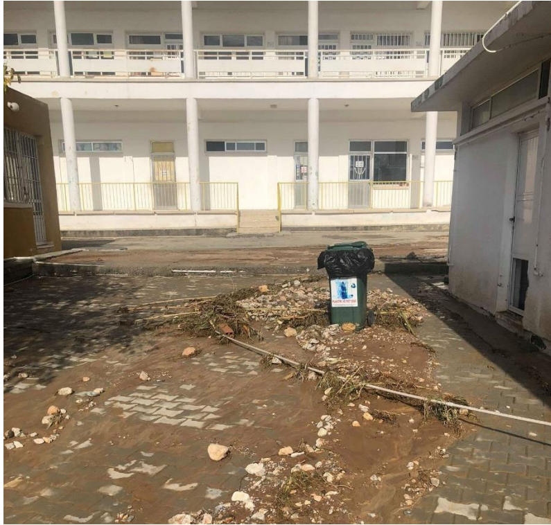
Figure 1.8 Dikmen Primary School After the 5 th December 2018 Flood (Cyprus-NEWS 2018)
